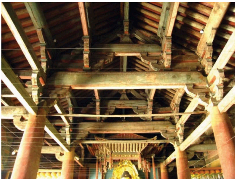
Figure 5. Interior timber frame structures of the Muryangsujön Hall.
