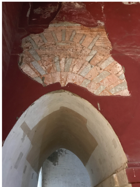
Figure 32. Bricks and stones masonry.
