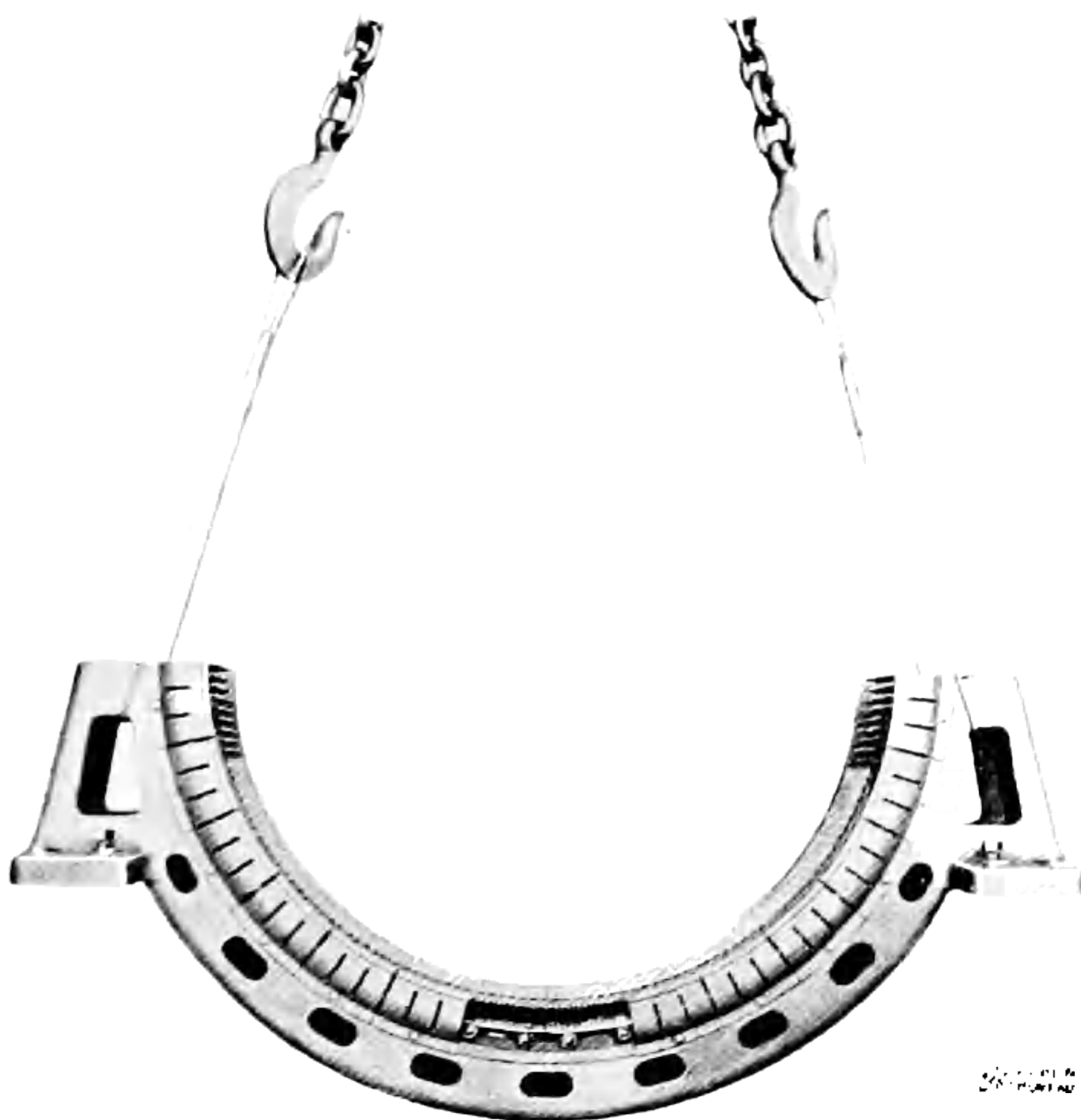
Fig. 24 METHOD OF LIFTING LOWER HALF OF STATIONARY ARMATURE WITH WINDINGS
