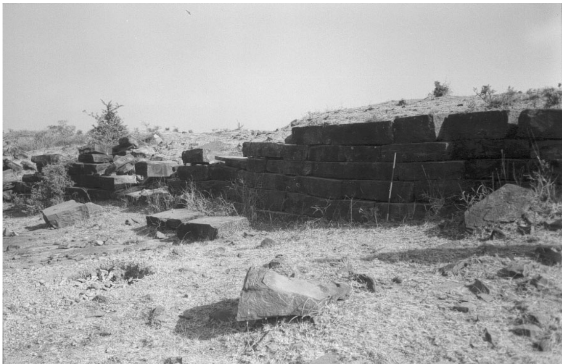
Fig. 4 Devrajpur dam: horizontally laid dam facing (after Shaw & Sutcliffe, 2001).
